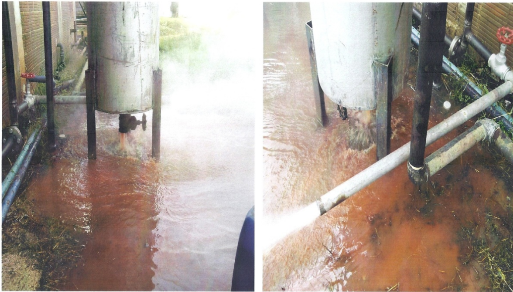
Ejected water runs red – the water contains suspended particles of rust that have dislodged from pipe walls.
